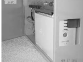
Battery System Status Indicators
